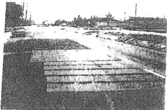
Reclamite was used as a construction seal on the dry areas of the pavement.
