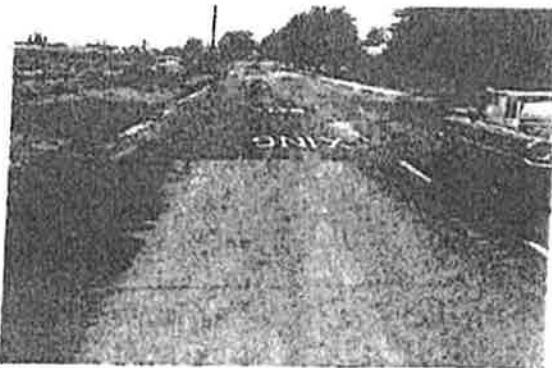
Reclamite was used as a construction seal on the dry areas of this pavement. Untreated areas are still wet from water penetrating the surface.
